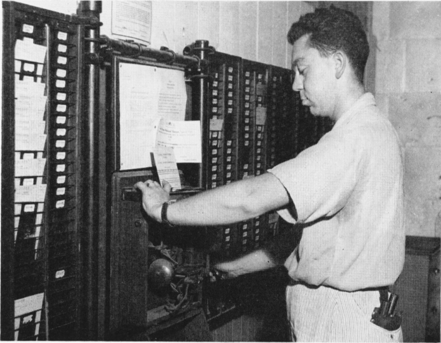
Harry E. Needham, Jr., of the Telephone and Signal Office, is checking the time on a time clock. Harry's is an out-of-the-ordinary job. It is quite important too, for it is necessary that time recorders be kept in time with the Master Clock.
